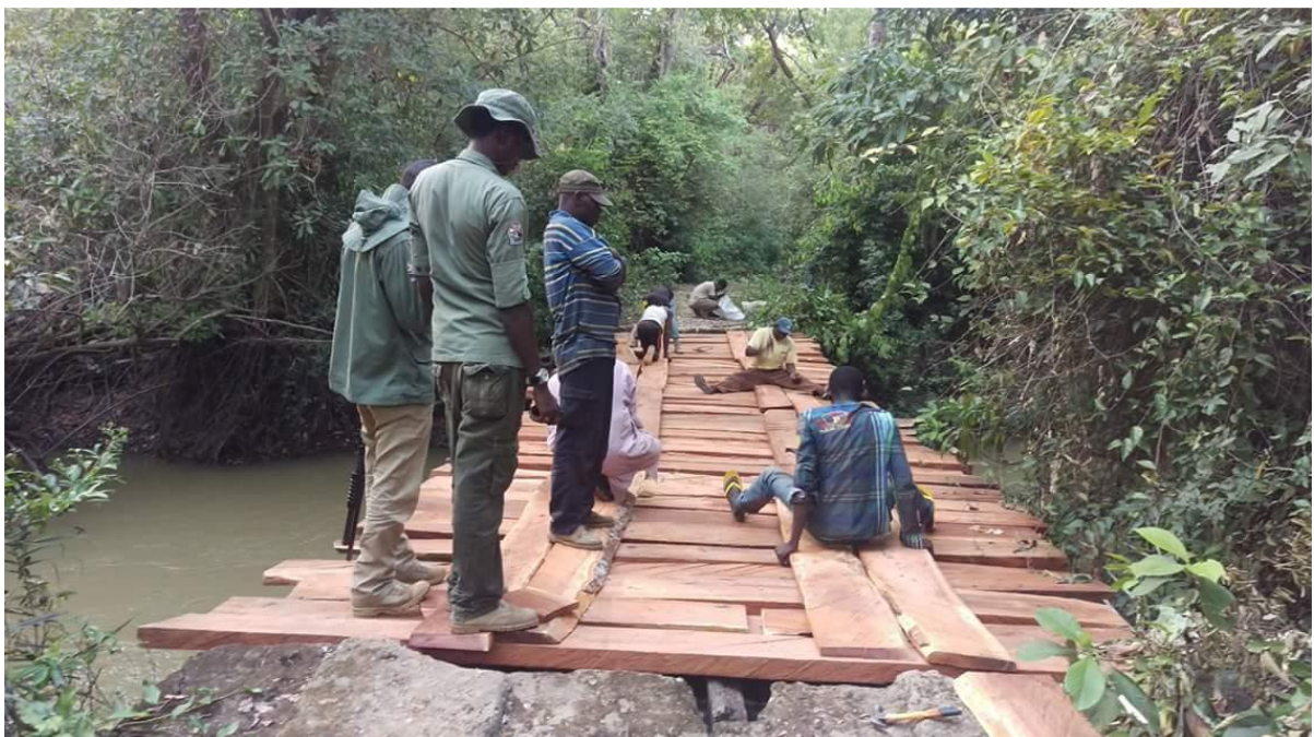
Guruntun Bridge in November 2015, fully repaired by WCS
