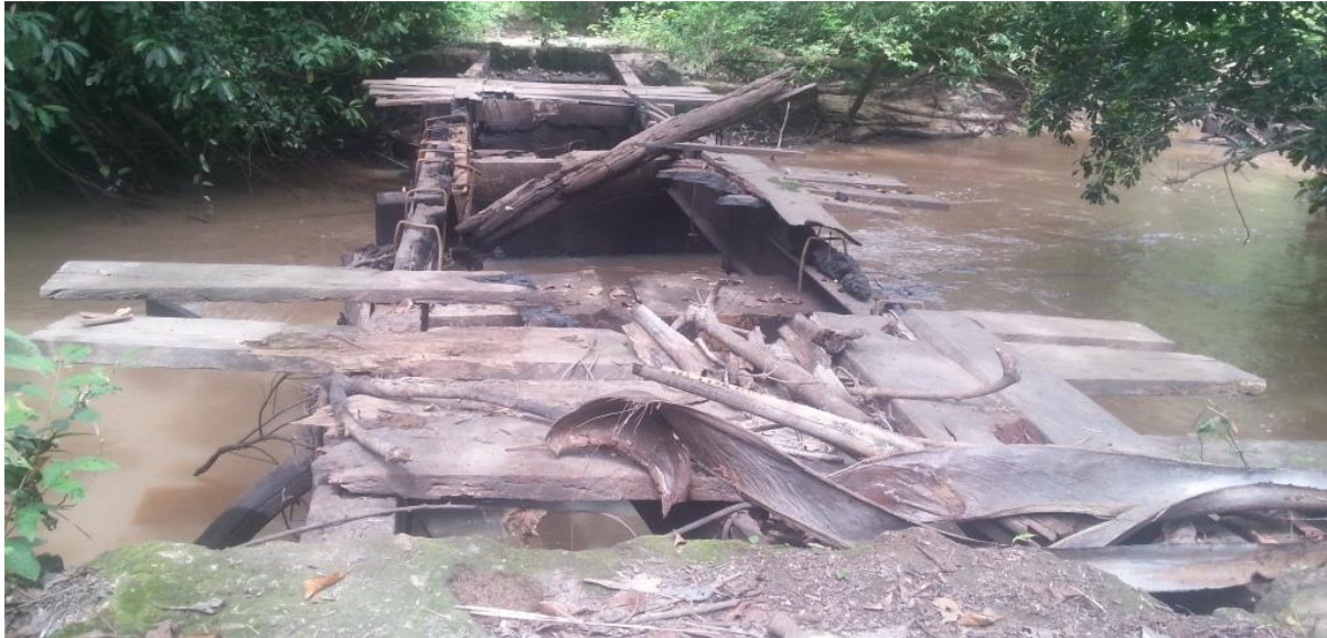
Guruntun Bridge in June 2015, destroyed by poachers.
